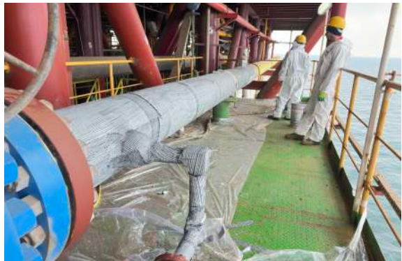
UMID 1 Gas Platform Passive Fire Protection (PFP) on live gas lines & valve jacketing (FR)
