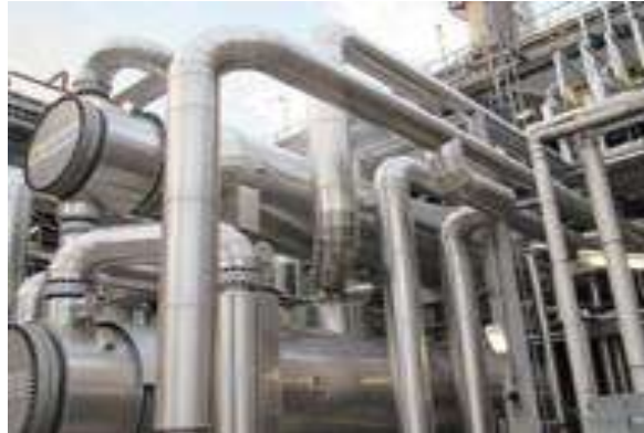
Insulation, Cladding & Heat Tracing
