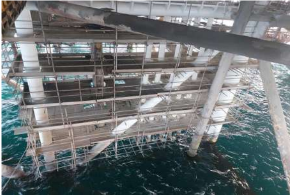
UMID 1 Gas Platform Blasting Painting of deck & jackets (legs)
