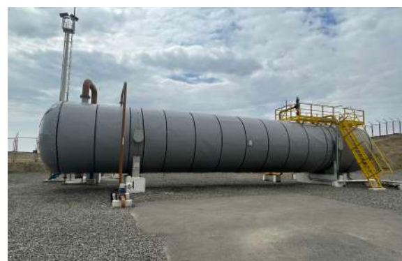
Pressure Vessel Insulation, Heat Tracing & Jacketing. Dashgil Gas Terminal
