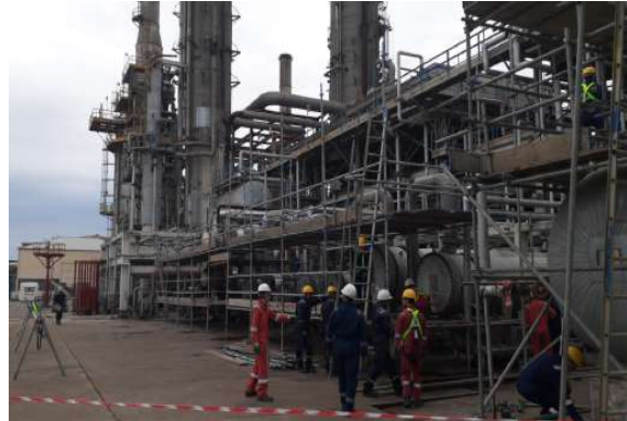
Shutdown / TAR Scaffold (150,000m3) HAOR Refinery TAR 2024
