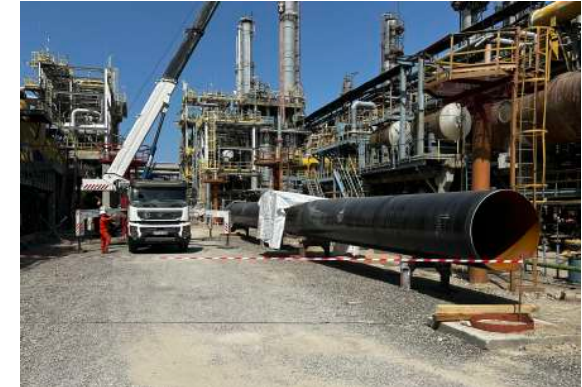
55" Pipeline, 2km long for Petrochemical Facility, Azerkimya PU
